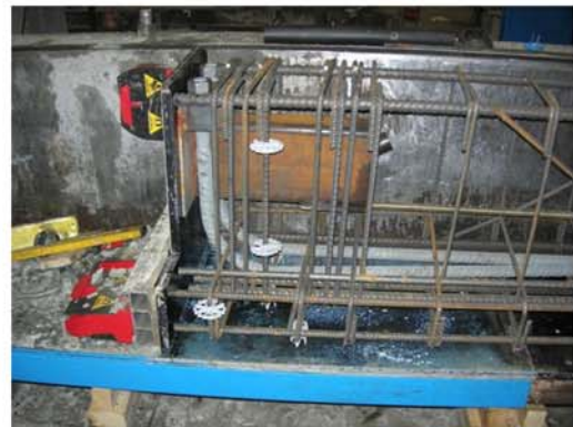
P16. BCC 450 is placed inside the reinforcement cage.
