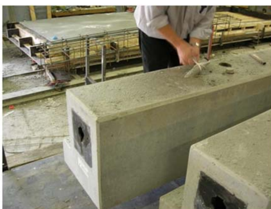
P23. Pull on the safety rope, until it's tight. Then tie a knot to the plastic tube.
