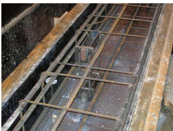
P9. Reinforcement of the column.
