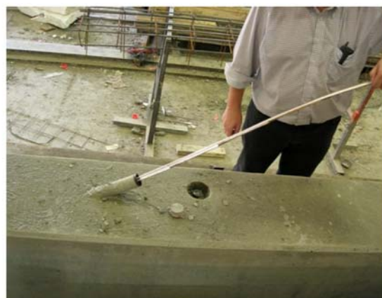
P20. Inserting the safety rope in the plastic pipe.
