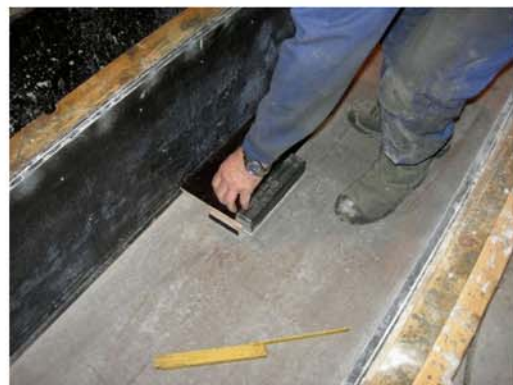
P6. Placing of the guiding unit for the column unit.
