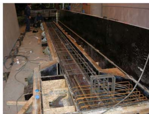
P10. The column is ready to be cast.
